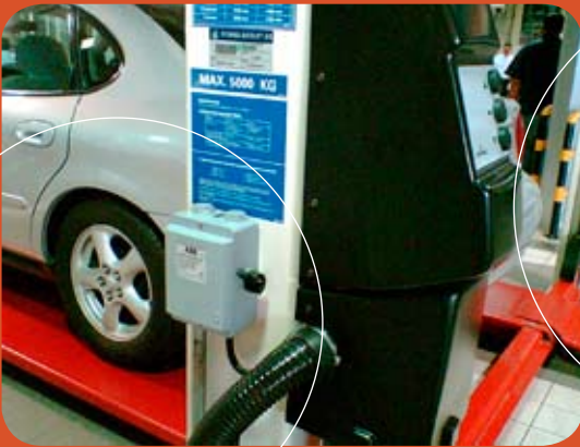
Aluminum enclosed side operated switch
