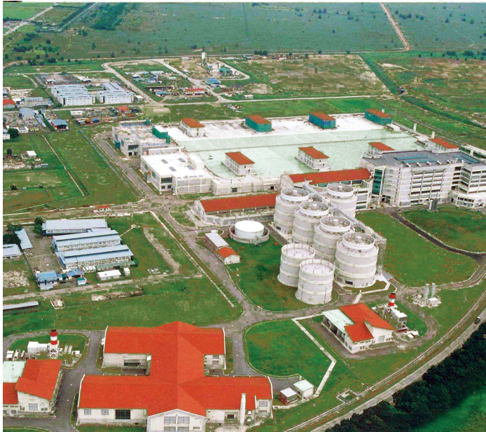
Source: Changi Water Reclamation Plant by PUB
