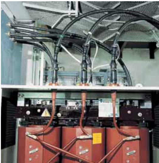
250 A HV plug-in bushings and separable connectors on IP31
